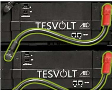
Install the remaining DC connecting cables (4.1) between the modules on the right side. Start with the bottom module.
