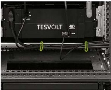
Fasten the cabinet connector cables in the bottom part of the cabinet to the cable retention rails (F) using cable ties. It is important to ensure while doing so that the cables are not crushed or damaged.
