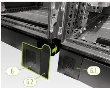
Now attach a left base corner cover plate (G.1) to the left corner at the front of the right half of the battery cabinet. Then you can attach the assembled cover plate to the right corner of the left half of the cabinet. Finally, fit the remaining base corner cover plates to the battery cabinet base's remaining corners.
