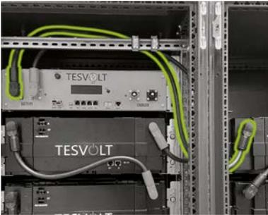
Connect the last module and the APU HV1000-S using the connecting cable (3.2). Make sure you follow the instructions in section "5.8 Wiring the battery modules" on page 24.
