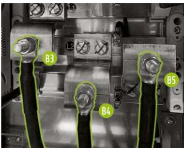
Now attach the AC connecting cables to the contact bolts B3 ... B5 of the busbars. Ensure that the phase conductors (L1 ... L3) are correctly assigned according to the markings on the busbars or section "9.2 TESVOLT PCS connection diagram" on page 49. The tightening torque is 70 Nm (secure the bolts against rotation using a spanner). Then reattach the touch guard. **Only with TN-C-S grid grounding type:** Please observe the following two installation steps before installing the touch guard.
