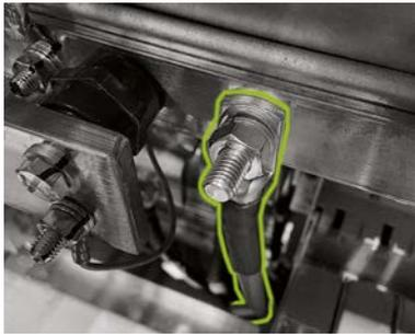
Now connect the grounding cable to the potential equalisation rail via the pre-assembled M10 or M12 contact bolts **51**. This is located immediately to the right of the N rail. The tightening torque is 40 Nm for M10 connections and 70 Nm for M12 connections (use a spanner to prevent the bolts from turning when tightening).
