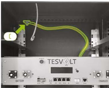
Attach the end with the M8 ring cable lug to the central grounding point (C). Use a torque wrench with a tightening torque of 10 Nm.
