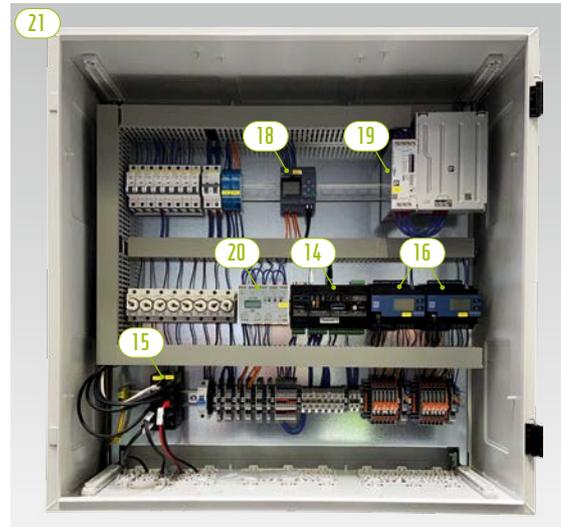
TESVOLT Backup Control Box with communication, measuring and control components
