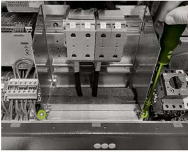
Loosen and remove the four screws that secure the DC connection bracket to the cabinet base.
