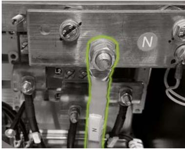
**Only with TN-C-S grid grounding type:** Now attach the N conductor to the N terminal **52**. Use a torque wrench with a tightening torque of 70 Nm (secure the bolts against rotation using a spanner). To simplify installation, remove the cable retention rail (perforated plate). Finally, reinstall the touch guard over the AC connections and lastly the cable retention rail.
