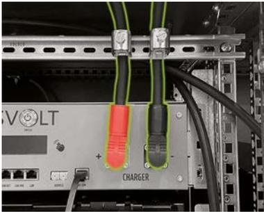
Only once connection of the TESVOLT PCS is complete, connect the DC cables (7.1) and (7.2) to the APU HV1000-S. **Please note that the plugs must audibly click into place.** Finally, fix the DC cables in the cable support clips (K).
