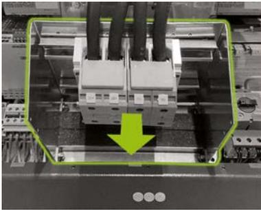
When all fastening screws have been removed, move the DC connector bracket toward the front of the cabinet so that you have adequate clearance in front of the AC connections.
