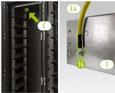
The APU HV1000-S must be grounded. Using the grounding cable (3.4), connect the APU HV1000-S to the central grounding point (C). To do this, first place the grounding cable's M6 ring cable lug onto the grounding bolt (14) (on the back of the APU HV1000-S) with a tightening torque of 6 Nm.
