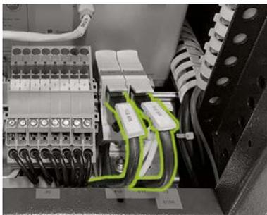
Connect the ethernet port **54** ① of the TESVOLT PCS with a network cable to connect the LAN 1 switch. Then connect a network cable to the Anybus port **54** ② of the TESVOLT PCS for the connection to the LAN 2 switch.
