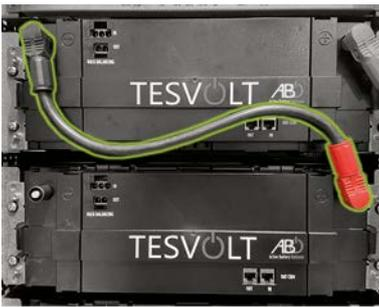
Then connect the remaining battery modules in this half of the cabinet with the DC connecting cables (4.1).
