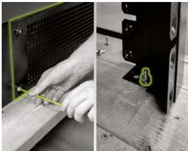
To lift the TESVOLT PCS off the transport pallet, the screw connections on the four feet of the control cabinet must first be removed. To do this, remove the base cover plates on at least two opposite sides of the base (front/rear or right/left). This is done by removing the screws at the corners of the plates. Now loosen and remove the screws at the feet of the cabinet.
