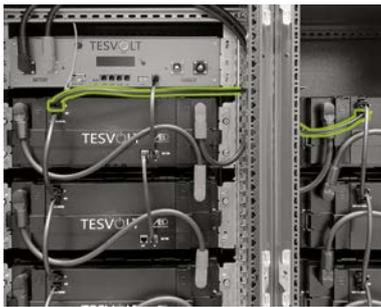
Now connect the remaining battery modules on the right side, starting from the bottom. Follow the instructions in section "5.8 Wiring the battery modules" on page 24. Finally, using the 0.75 m rack balancing cable (6), connect the rack balancing "OUT" connection of the top module on the right half of the cabinet to the rack balancing "IN" connection of the top module on the left side.
