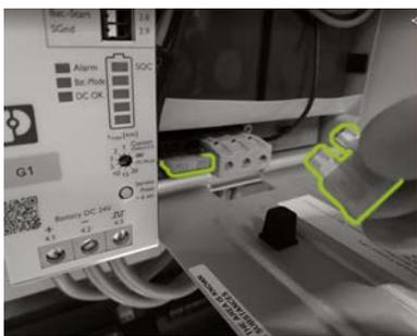
First activate the UPS 93. First open the battery housing and insert two 25 A blade fuses into the slots provided.
