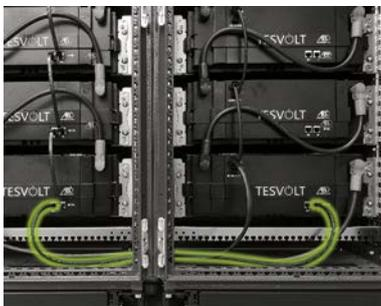
Establish the BAT-COM connection between the bottom battery modules using the longer patch cable (5.2). Next, connect the remaining modules in the right half of the cabinet, starting at the bottom and using the patch cables (4.2). The last battery module's BAT-COM "OUT" connection remains open.
