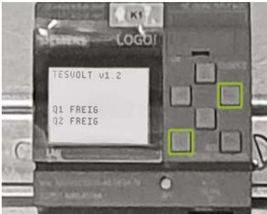
Now close the grid disconnection switches. This will apply voltage to the system. The basic prerequisite for this is that the TESVOLT PCS is inactive/idle and that no other off-grid system is formed (e.g. by way of a diesel generator), i.e. that the customer grid is voltage-free on the AC side. To close the grid disconnection switch, simultaneously press the (ESC) + (→) keys on the SIEMENS Logo <sup>92</sup> controller.
