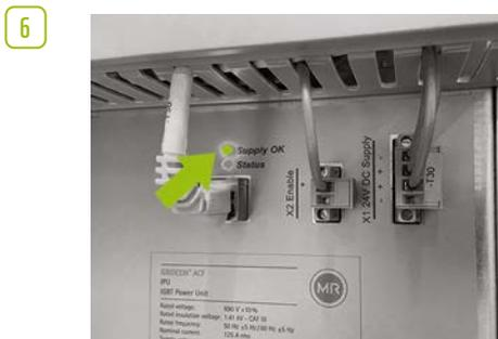
Close the main switch S1 (23). First, the fans of the TESVOLT PCS are tested. After successful completion of the selftest, the upper "Supply OK" LED on the IPU(s) lights up green and the TESVOLT PCS is in operation.
