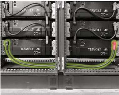
Connect the bottom two battery modules using the long DC connecting cable (5.1) from the cabinet connector set (5).
