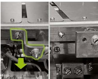
**Only with TN-C-S grid grounding type:** Before installing the N conductor connection, remove the bridge B6 between the PE rail and N rail.
