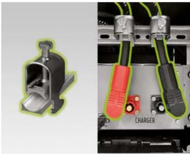
Now lay the DC cables (7.1)/(7.2) starting from the APU HV1000-S "CHARGER" (12)/(13) to the TESVOLT PCS. The red plug is intended for connection to the positive pole and the black plug for connection to the negative pole. Please note that the cable can only be shortened on the TESVOLT PCS side. To relieve the strain on the DC cables, install the two cable support clips (K) above the CHARGER connections of the APU HV1000-S (I) on the C-rail (D).
