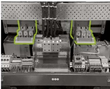
Before connecting, make sure that all fuse switch disconnectors Q1 ... Q4 (28) are open (according to the number and positioning of the IPU) and switch S1 (23) is set to the "OFF" position.
