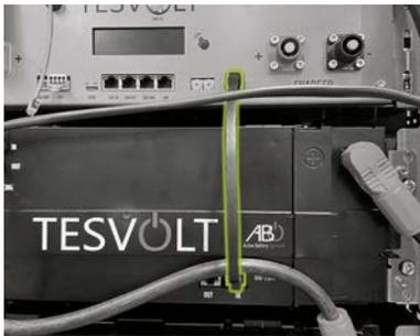
Connect the BAT-COM communication cable using the supplied patch cables (3.3) and (4.2). Connect the "BAT-COM" (11) connection of the APU HV1000-S and the BAT-COM "IN" connection of the battery module positioned below the APU HV1000-S using a patch cable (3.3). Then use a patch cable (4.2) to connect the same module's BAT-COM "OUT" (73) connection to the next module's BAT-COM "IN" (74) connection.
