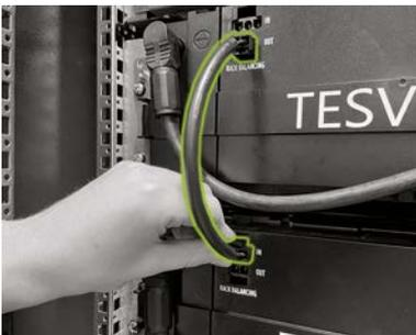
Connect the rack balancing "OUT" connection (2.2) of the first battery module below the APU HV1000-S to the rack balancing "IN" connection (2.1) of the next battery module down using a rack balancing module connector (4.3). Continue in this manner, connecting all the battery modules in the left half of the cabinet.
