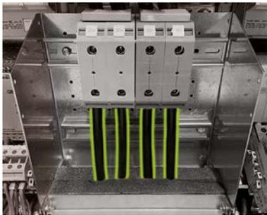
When installing the DC connection of the battery, make sure that the polarity is correct. The tightening torque is 6–8 Nm.
